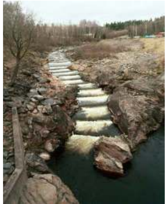
Figure 7. Fish pass in Söderhamn, 4 m drop, 80 m bypass and Gullspangsalven, steep pool
