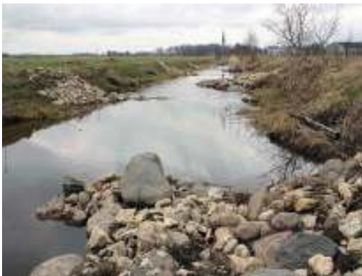
Figure 19. Measures in dredged rivers, stone deflectors (left) and stone weir (right)
