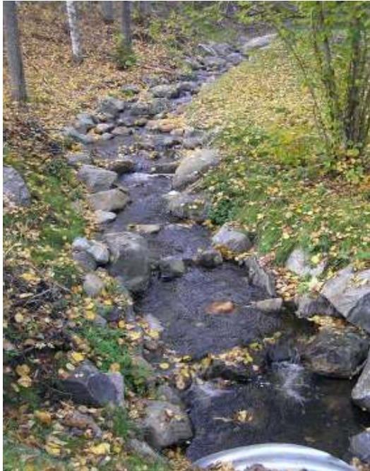
Figure 7. Fish pass in Söderhamn, 4 m drop, 80 m bypass and Gullspangsalven, steep pool
