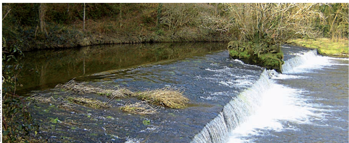
The weir of the Houël mill, in 2010 prior to the works.
