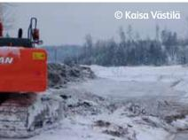
A flood terrace was built on the left hand river bank. The right hand river bank was left untouched. Soil dug for the flood terrace was used on nearby fields.
