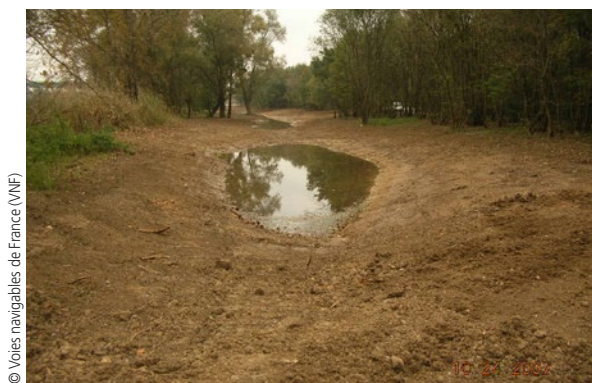
Earthwork to restore a side channel and ponds. October 2007.
