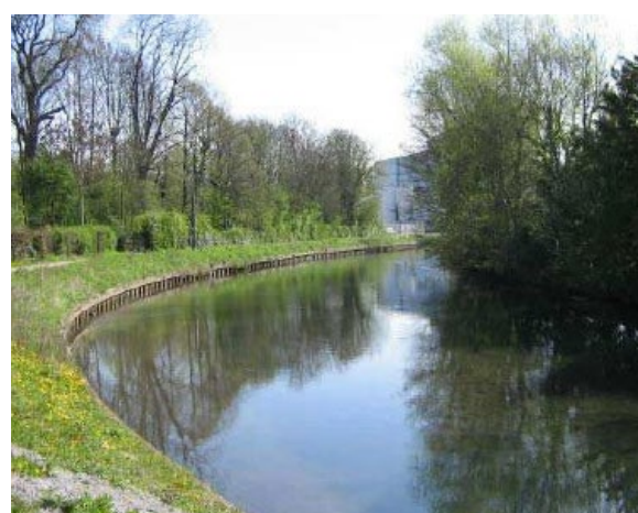
Banks protected by sheet piles prior to the restoration works. Autumn 2010.
