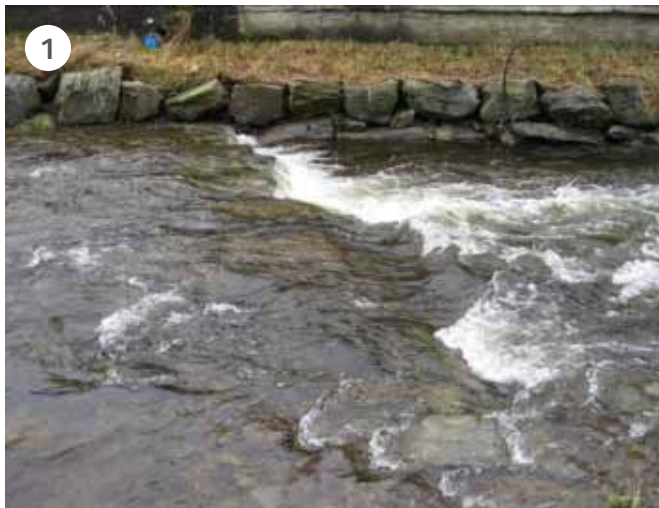
(1) Blockstone check structure preventing upstream erosion, (2) Bar forming on right-hand bank.
