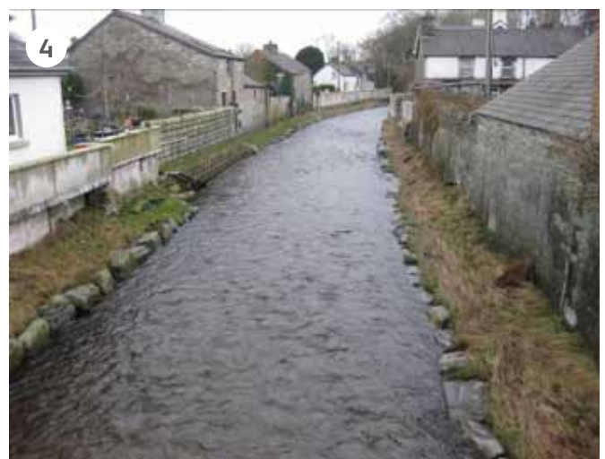
(3) Rock and geotextile revetments and a blockstone check structure at the upstream end of the regraded reach; (4) Rock and geotextile revetments on both sides of the channel.
