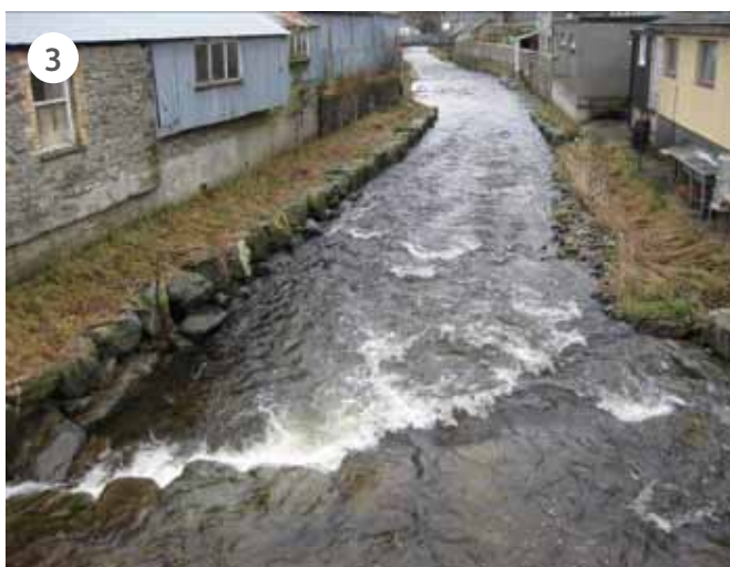
(3) Rock and geotextile revetments and a blockstone check structure at the upstream end of the regraded reach; (4) Rock and geotextile revetments on both sides of the channel.
