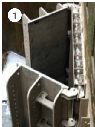
(1) Gate at Ashlone Wharf;
