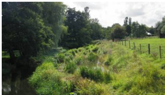
Post-restoration channel - berm feature installed to narrow channel. Courtesy of the River Restoration Centre.
