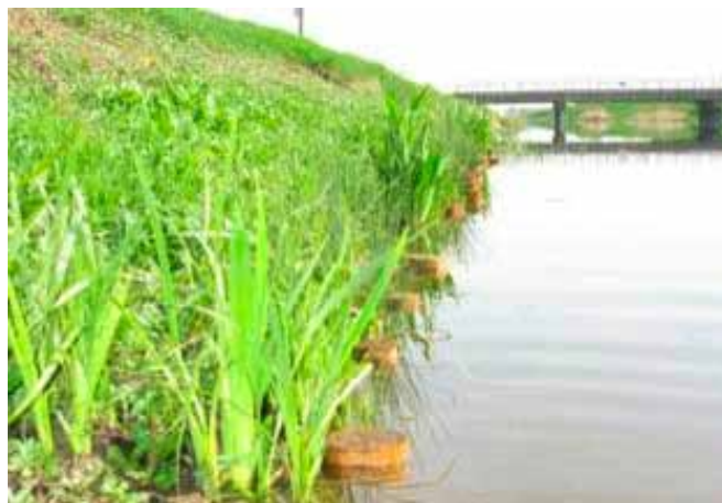
April 2009, three months after installation, yellow flag is the first plant to develop. Summer water level is now nearly covering the coir rolls.
