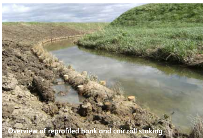
1) Failing bank at Cottenham, before scheme implementation 2) Installation of "soft" bank protection
