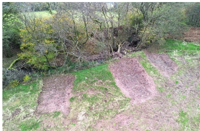
FIGURE 4 Embankment removal and large wood structure behind. © NRW
