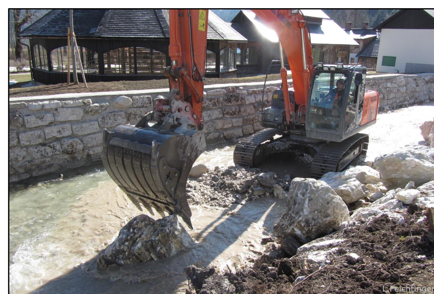
Fig.3: Restructuring river bed after flood protection measurments.
