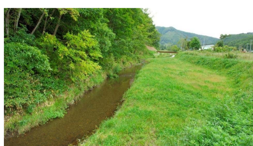
One-side widening for conservation and cost reduction
