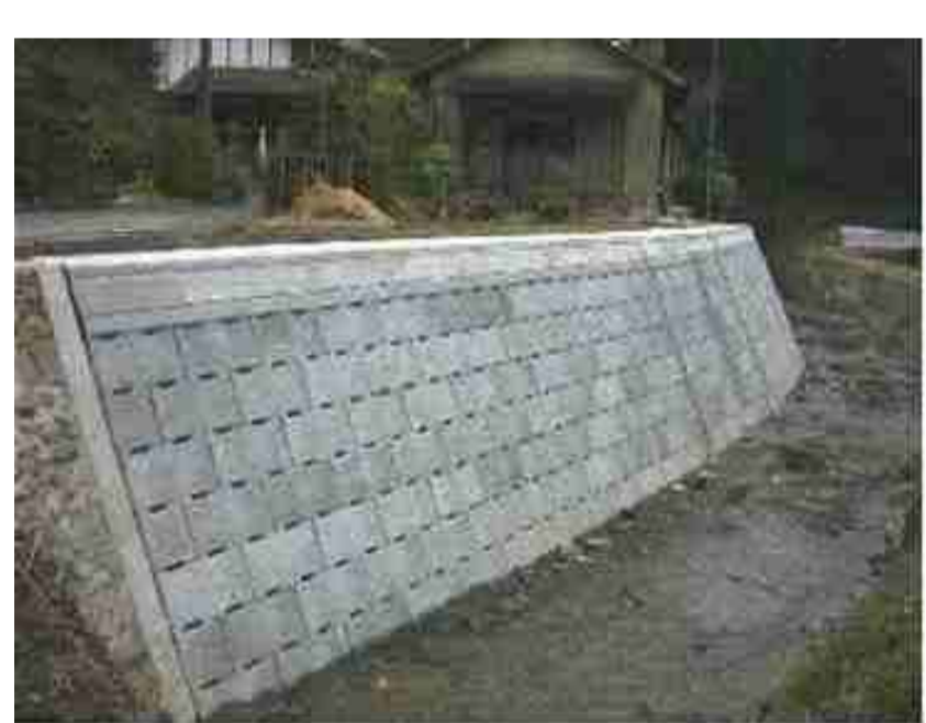
Post-disaster works tend to use concrete block (image)
