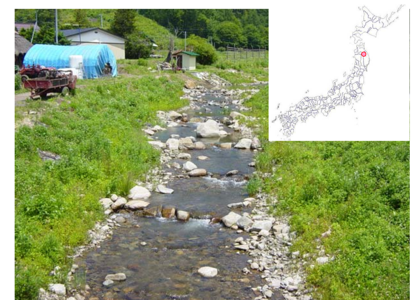
Covering the revetment for better landscape and allowing ecotone dynamics
