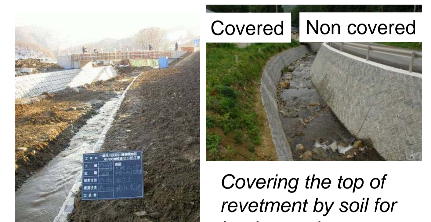
Covering the revetment for better landscape and allowing ecotone dynamics
