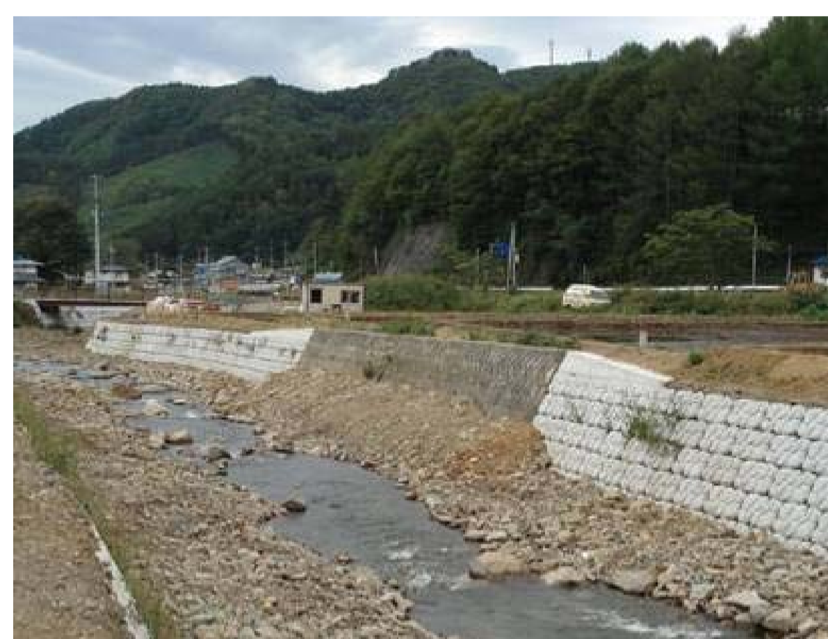
Partially covering the revetment for better landscape and ecotone with vegetation
