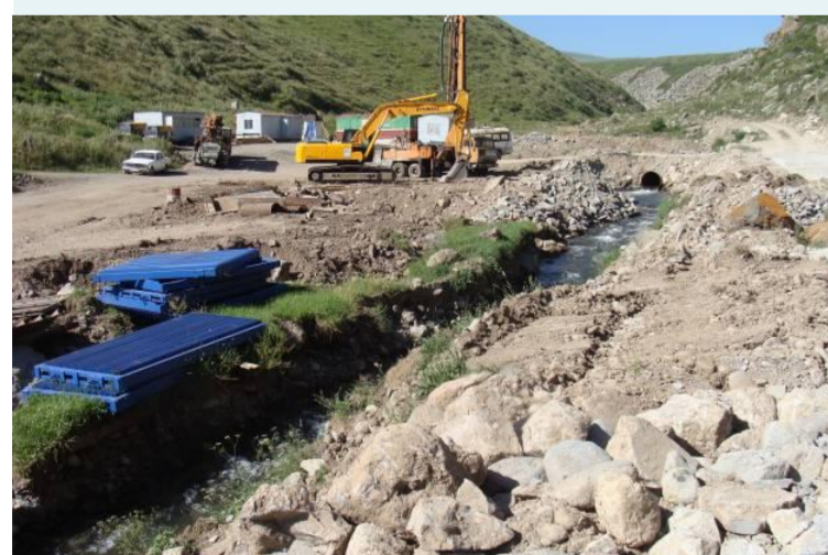
Construction of HPP on river Vardenik.
