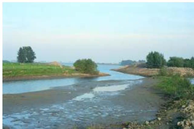
Figure 19. Example of a natural flood risk reduction measure: a reconnected side channel Photo: Grontmij
