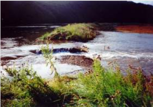
Figure 55. Breaching – the construction of breaches in the embankment allows water to flood the site at high tide
