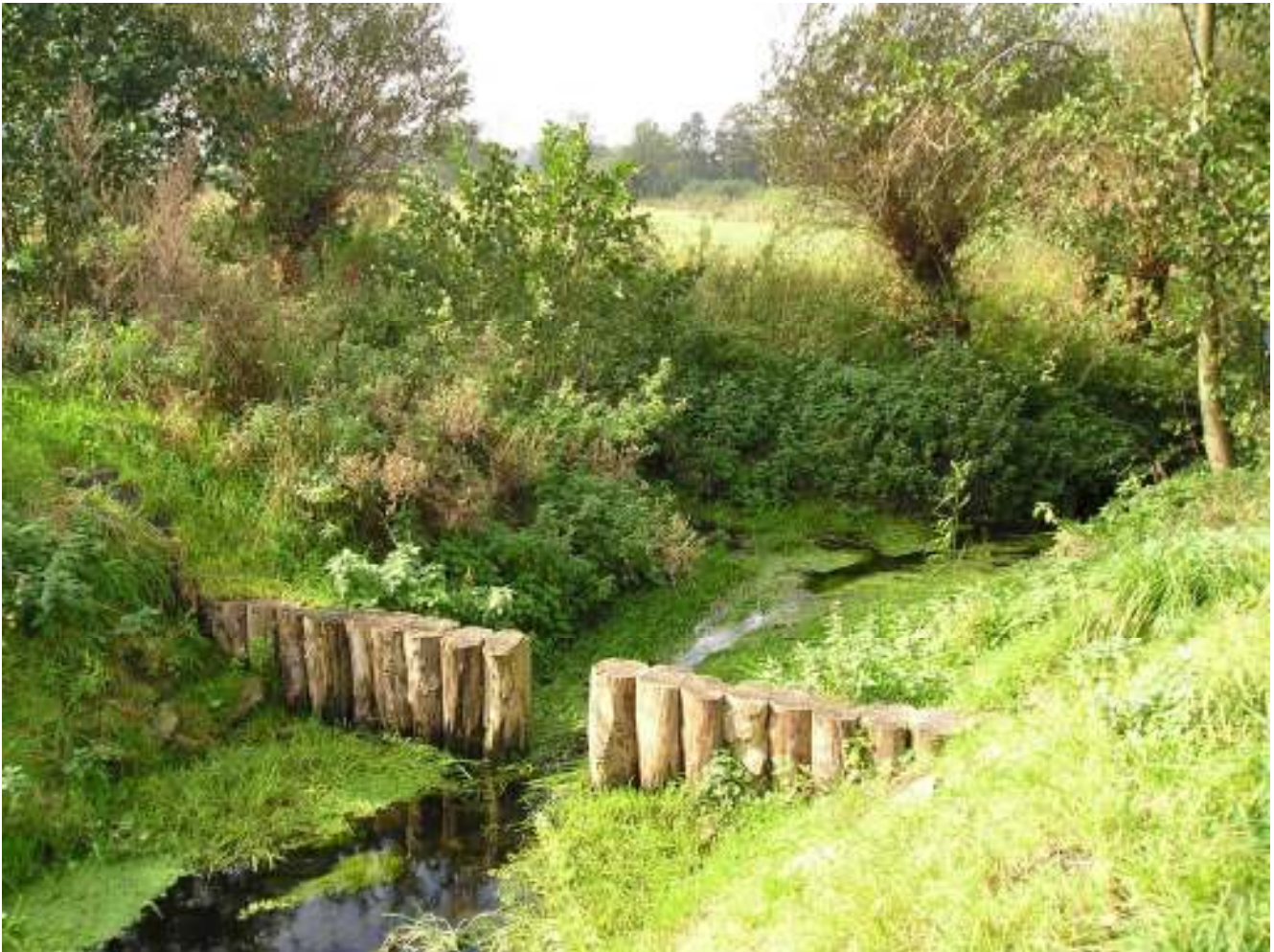
Figure 14. Retaining water in headwaters as a runoff reduction measure Photo: Y. Wessels/Grontmij
