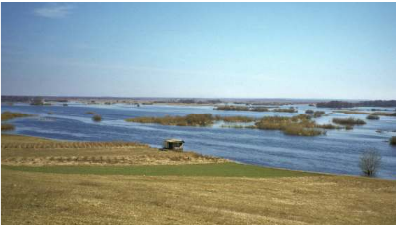
Figure 24. The Biebrza River Valley, Poland, storing water during a flood event Photo: T. Okruszko/SGGW
