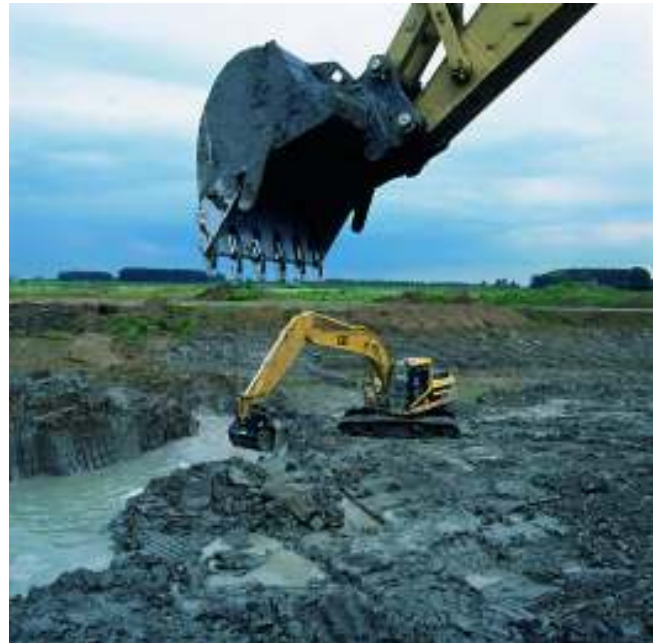
Figure 16. Lowering the floodplain provides more storage for flood water. Photo: Grontmij
