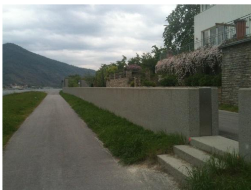
Oberarnsdorf: Fixed base of the flood wall, Danube cycling route and flood 2013 © Zinke, Hydro Ingenieure
