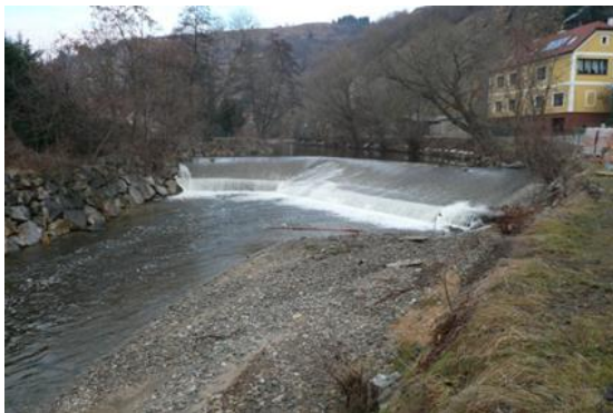
Krems river sites before and after re-building and restoring the urban river bed; guided by a new flood wall. The bottom weirs are replaced by rocky structures facilitating fish migration. © Hydro Ingenieure
