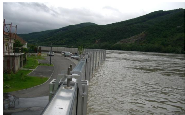
Oberarnsdorf: Fixed base of the flood wall, Danube cycling route and flood 2013 © Zinke, Hydro Ingenieure
