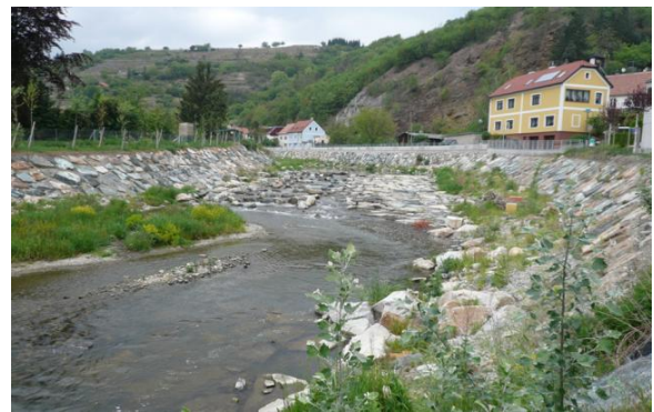
Krems river sites before and after re-building and restoring the urban river bed; guided by a new flood wall. The bottom weirs are replaced by rocky structures facilitating fish migration. © Hydro Ingenieure
