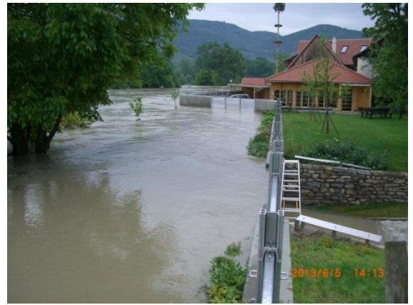
Rührsdorf: new combined flood wall at the June 2013 flood © Hydro Ingenieure
