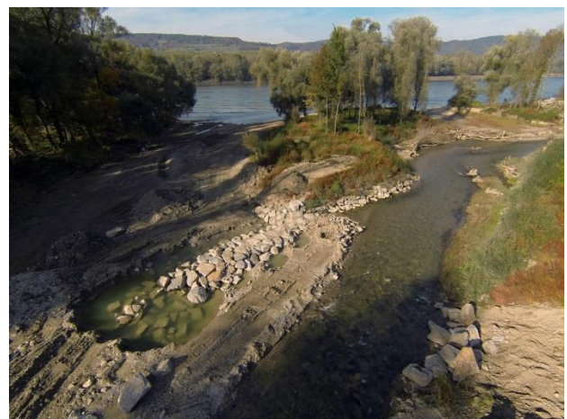
Rebuilt mouth of Pielach river restoring the
