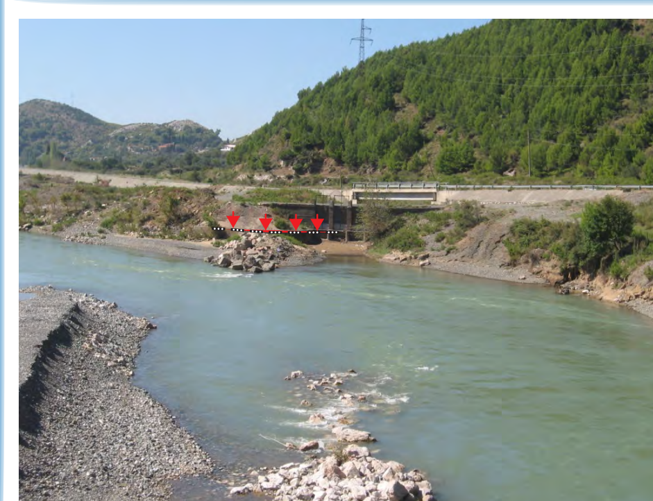
Irrigation Infrastructure on Mati river out of work
