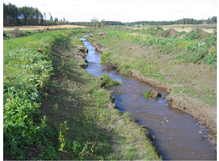
Juottimenoja brook in Southern Finland before and after environmentally friendly dredging
