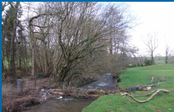
Woody debris installed in Belford Burn
