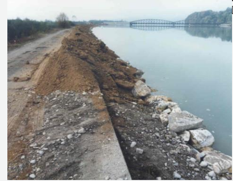
Binding soil layer on gravel
