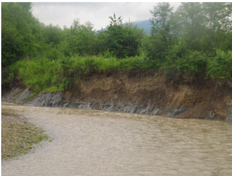
Landslides and erosion are a problem e.g. at Biala River in Southern Poland.
