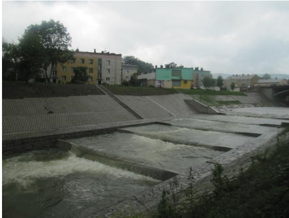
Recently finished fishway at Grybow, Southern Poland. The fishway seems functional, but could be made of natural stones to maximize the benefits for fish and landscape (see right hand side photo).
