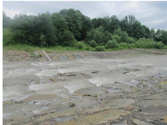
Recently finished fishway at Grybow, Southern Poland. The fishway seems functional, but could be made of natural stones to maximize the benefits for fish and landscape (see right hand side photo).
