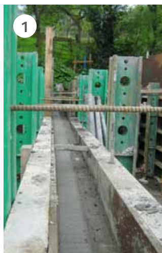
(1) Concrete U-channel of the fish pass during construction; (2) U-channel once completed
