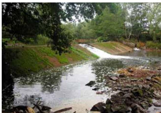
(1) Kentchurch weir during high flows; (2) Kentchurch weir during low flows, just prior to removal
