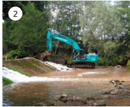
(1) Straw bales in place as a downstream sediment trap; (2) Excavator lowering the first section of weir to create a flow channel; (3) Demolition of the main weir; (4) Earthworks to previous site of weir after
