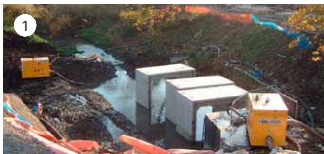
(1) Culvert at the Moselle Brook during construction; (2) the newly-restored channel after construction.
