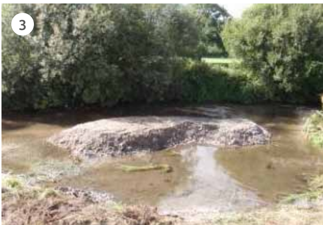
(1) Bed reprofiling; (2) Bank reprofiling; (3) Riffle creation; (4) Bed raising
