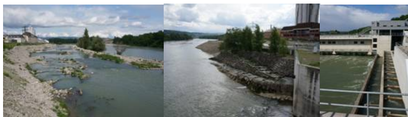
Left photo: Rheinfelden fish pass facility. Middle photo: a rock cascade pass. Right photo: a vertical slot pass (photos by Sini Olin, SYKE).
