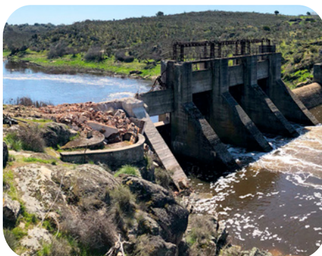
Yecla de Yeltes dam during removal © Herman Wanningen WFMF
