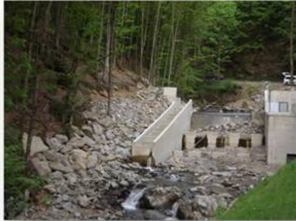
Fish ladder from MHC on Valea Bistra, Barcau, b.h. Crisuri (photo: G. Petrescu, 2013)
