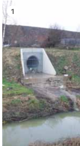
1) View of outfall before works
