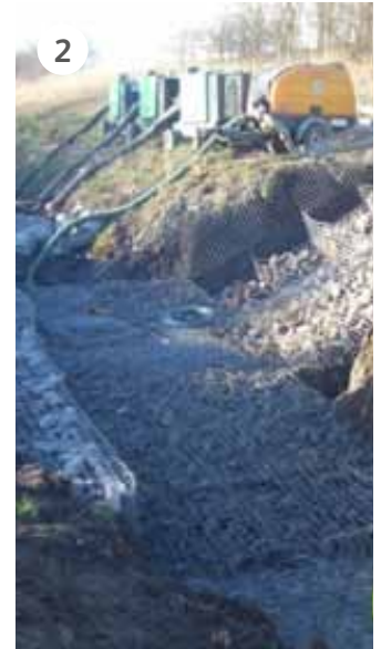
2) Reinforcement with stone gabions
