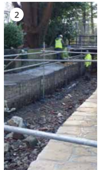
(1) Lowering of the existing weir; (2) Installing gabion baskets in dry-working area behind clay-bunds
