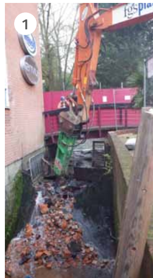
(1) Lowering of the existing weir; (2) Installing gabion baskets in dry-working area behind clay-bunds
