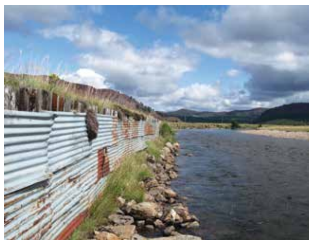
Figure 3.4 (Above) Bank reinforcement to stop natural erosion constructed from boulders on the Ewes Water, Dumfries and Galloway (© Martin Janes, RRC) and (Below) using corrugated iron and rubble on the River Dee, Aberdeenshire, Scotland. The River Dee bank reinforcement was removed in October 2015 to improve connectivity with the floodplain (© James Hutton Institute).
