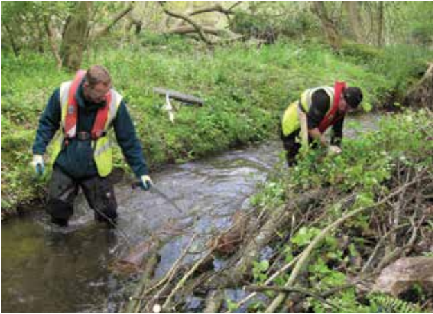
Figure 5.10 (Left) Wood placement in the River Wensum catchment, Norfolk to diversify river habitats (© Adam Thurtle, Environment Agency). (Right) One year after the placement of wood to diversify river habitats on the Allt Lorgy, Highland (© Liz Henderson, Spey Catchment Initiative).
