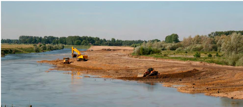
Existing gravel pits were integrated into the river system by lowering the banks.
