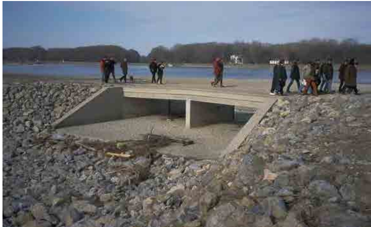
Fig. 7. The Danube restoration programme at Regelsbrunn, a first decisive step. Restoring the lateral connectivity between the river and the floodplains by lowering the inflow areas, construction of lateral weirs and enhancing the longitudinal through-flow in the side arm system (a). A photograph of an inflow area (b). After Schiemer et al. 2006
