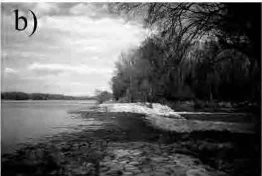
Fig. 7. The Danube restoration programme at Regelsbrunn, a first decisive step. Restoring the lateral connectivity between the river and the floodplains by lowering the inflow areas, construction of lateral weirs and enhancing the longitudinal through-flow in the side arm system (a). A photograph of an inflow area (b). After Schiemer et al. 2006
