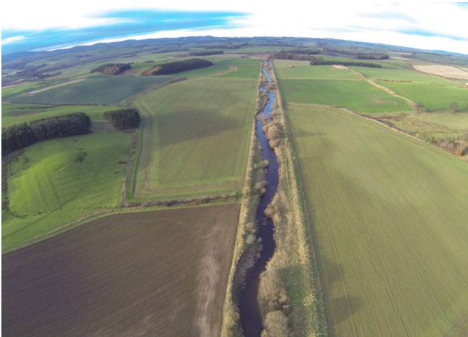
FIGURE 2 River Breamish before restoration. Credits: Tommy Wilkinson.
