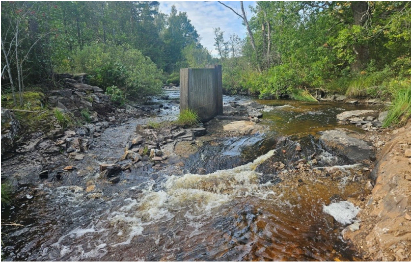
FIGURE 2 Section of the barrier that was removed and the braided river system downstream was activated again. © Ebbe Berglund
