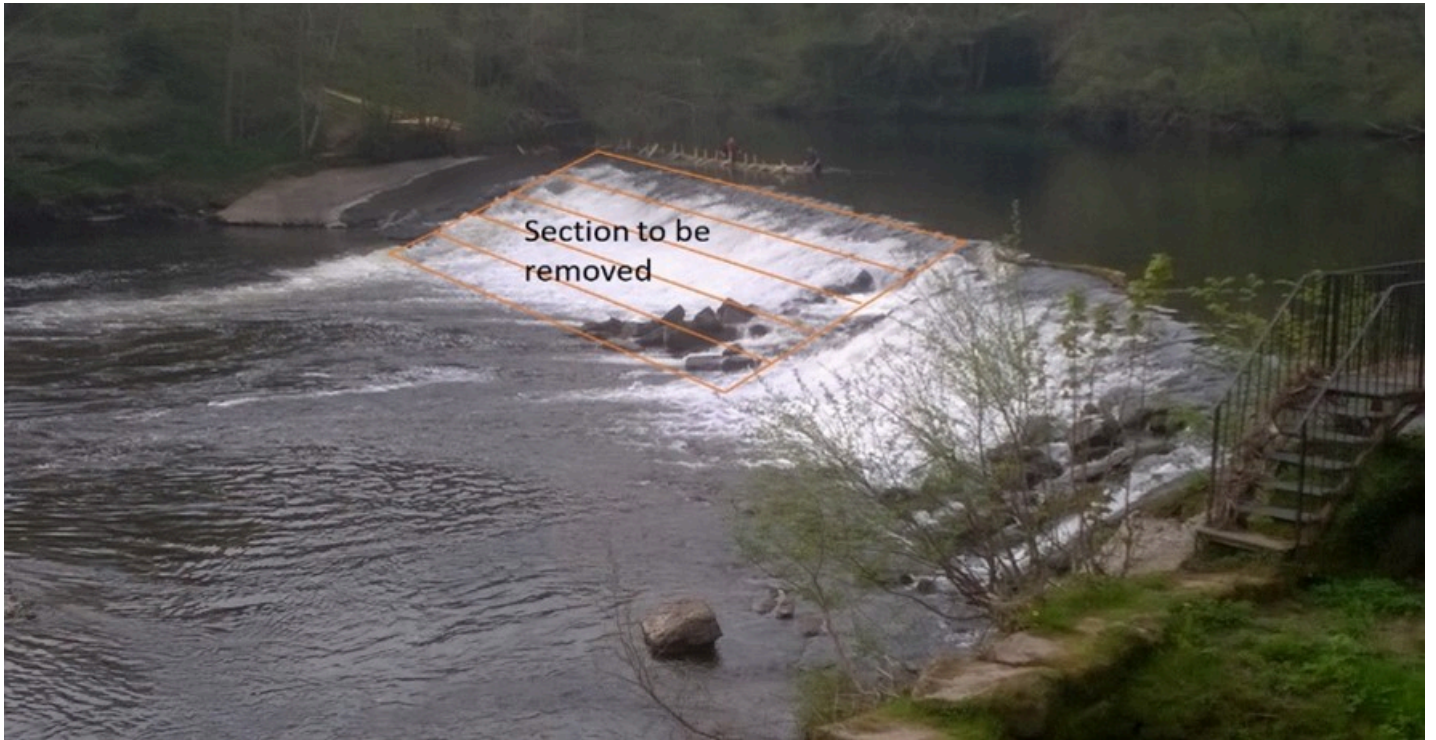
FIGURE 2 Side view of section to be removed taken from lefthand bank till current damage to weir face. © LIFEDeeRiver
