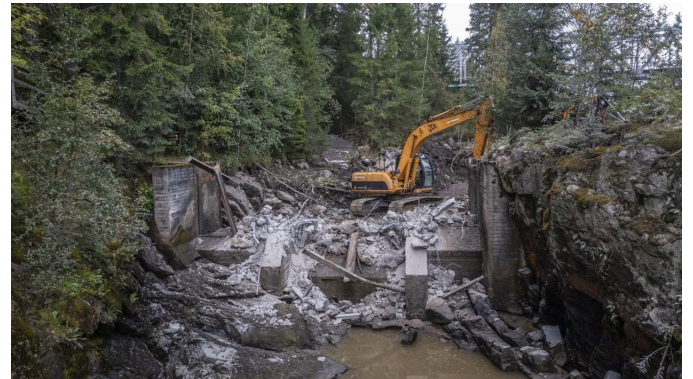
FIGURE 7 Finland Ritaksoki dam during removal. Credits: Mikko Nikkinen.
