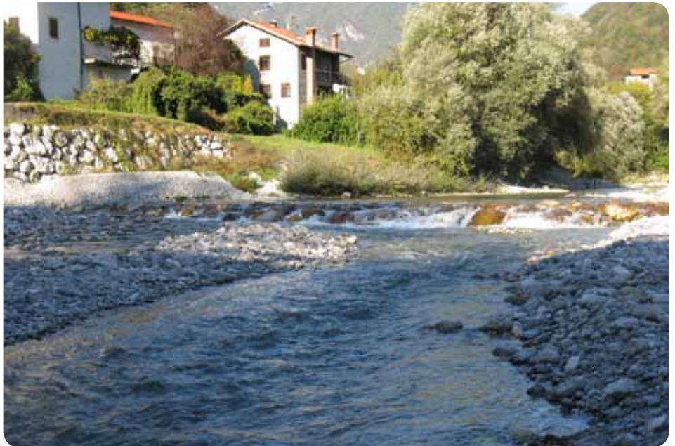
River restoration on the Bača River - dam removal (Photo: M. Habinc)
