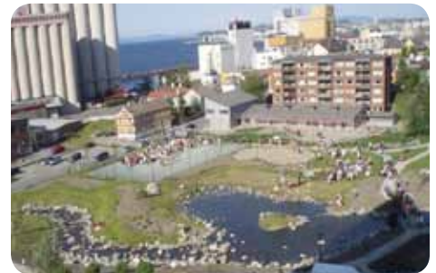
reopening of urban river stretch at Ila in Trondheim city, 70 years after it was enclosed in underground tubes. (Terje Nøst, Trondheim Municipality).
