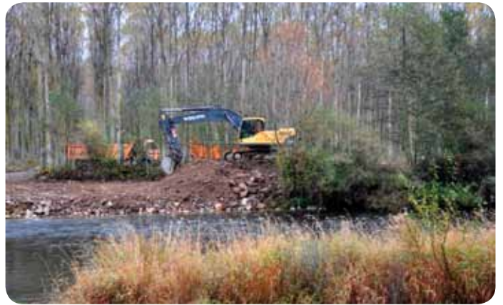
Works to eliminate earth embankments in stretch I of the ecological improvement project in the Órbigo River and orthophoto of a portion of the stretch showing the earth embankments that are eliminated and/or moved away from the channel
