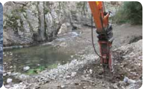
Finalization of the work
