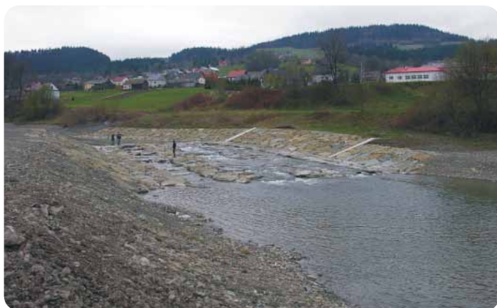
A fish pass on the Biała Tarnowska River constructed in the place of a dismantled weir.
