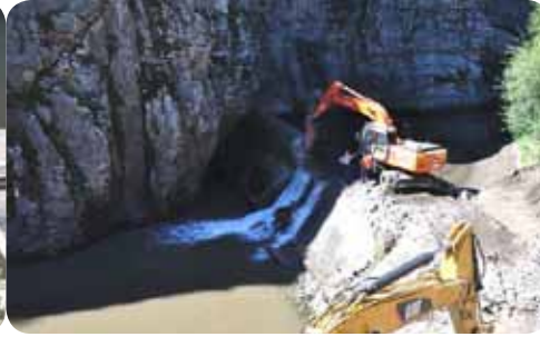
Demolition of the wall starts
