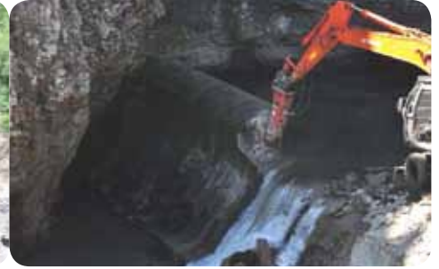
Detail of the demolition of the wall
