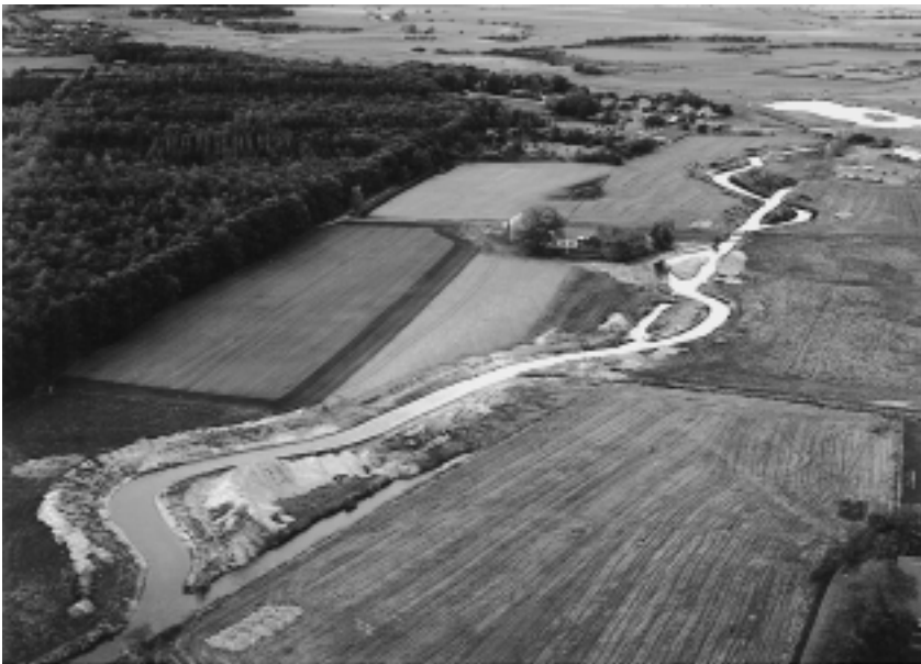
Figure 2. The River Brede near Løgumkloster during restoration. The new meanders have been dug and the former channelized path has not yet been filled in.
