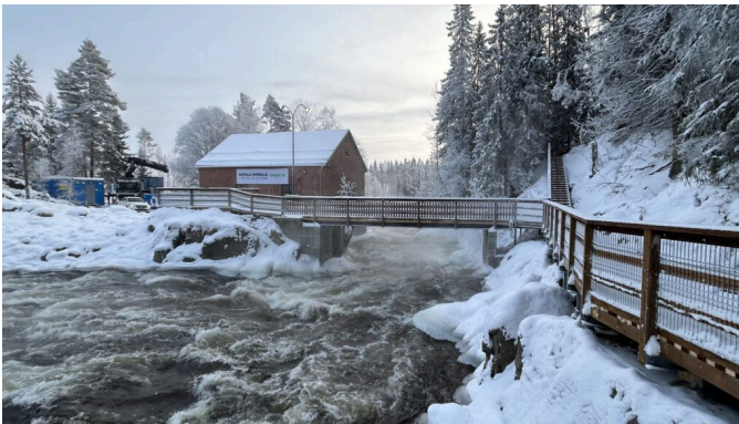
FIGURE 2 The upmost dam of the river Hiitolanjoki at the Ritakoski power plant was opened
