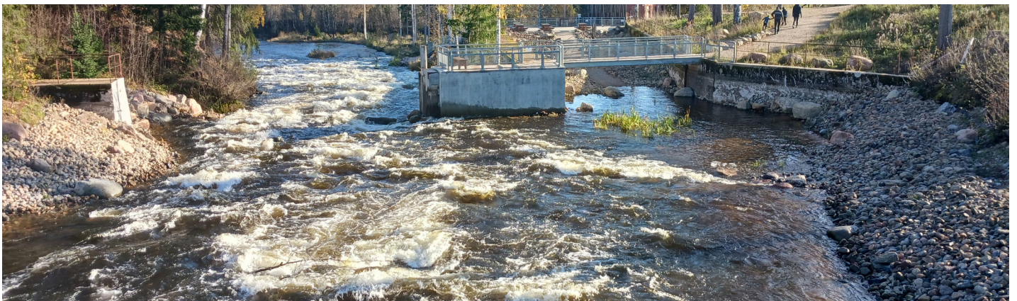
FIGURE 4 The restored Kangaskoski rapid with the opened dam
