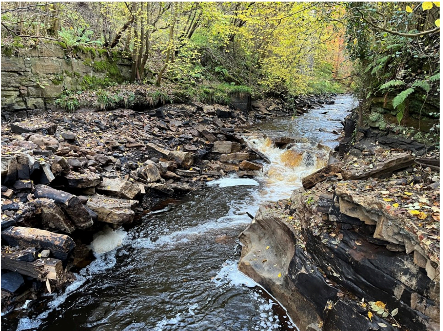
FIGURE 4 Weir removed and gravels washed down after autumn storms. Now fully accessible.
