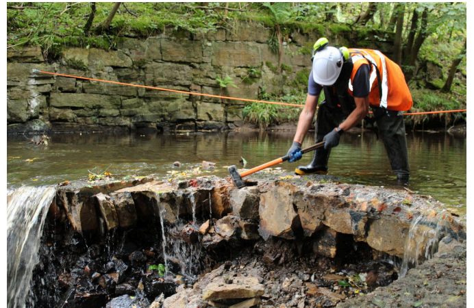
FIGURE 2 Scot Muir using a sledge hammer to remove coping stones from the weir.
