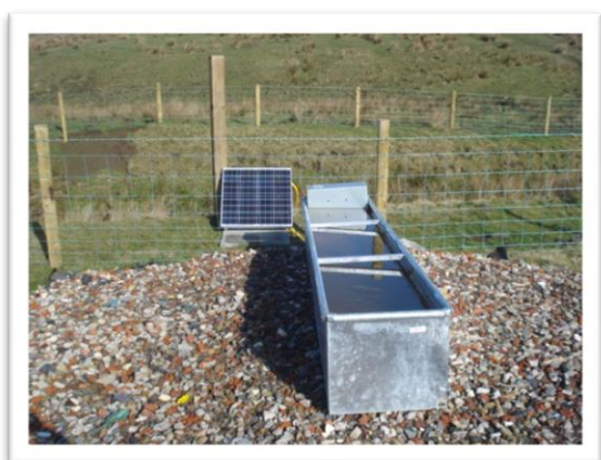
Figure 14. Solar powered stock watering trough in the Ribble catchment (Photo provided by Jack Spees, Ribble Rivers Trust Director)
