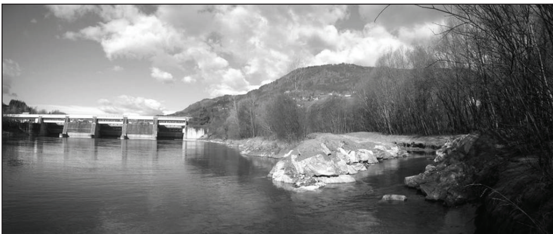
fish pass channel entrance
