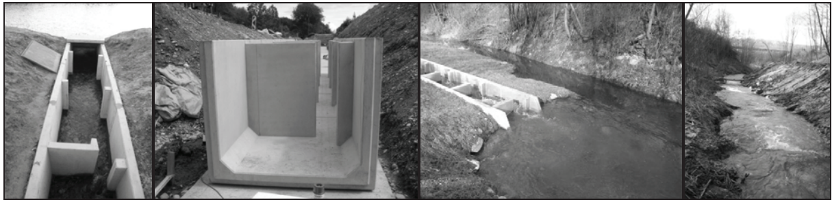
Vertical slot fishpass and natural bypass channel section.
