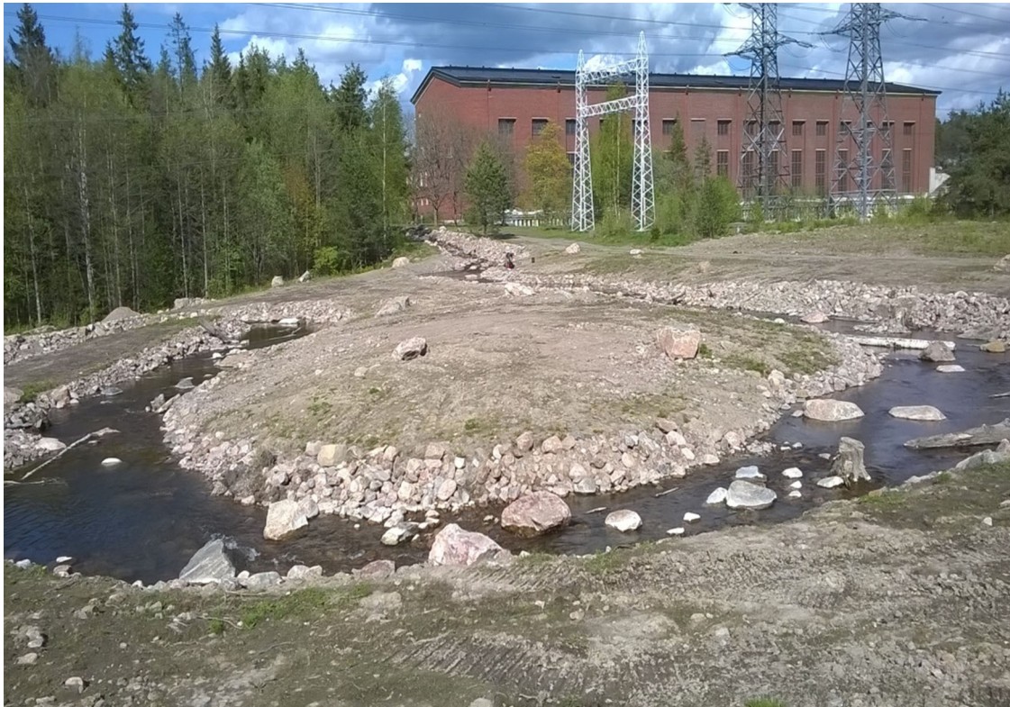
Figure 3. The habitat section was designed with a winding channel and small gradients, with deeper pools in between.
