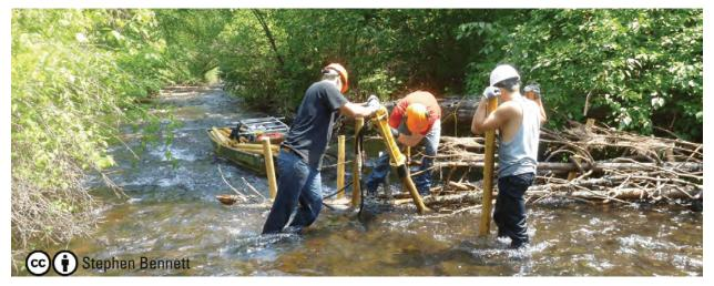
Figure 8 – A crew of three building a post-assisted log structure.
