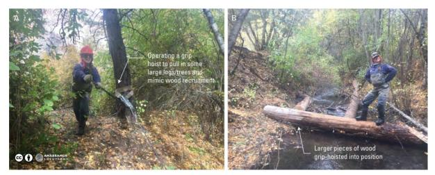
Figure 16 - Example of using a grip hoist to pull in wood into the riverscape (i.e. mimicking process of wood recruitment) to enhance or create a new wood accumulation (structure) in treatment sections as part of ongoing treatments until the processes of wood recruitment and wood accumulation are self-sustaining.
