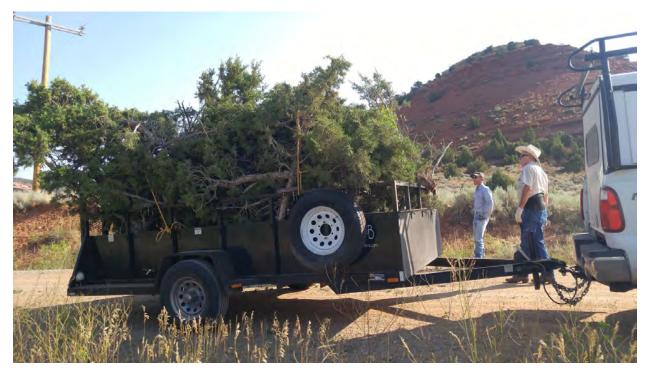
Figure 14 – Low-tech restoration is primarily about getting structure (e.g., wood, branches, logs, trees, sticks, posts) back in riverscapes. To add large amounts of structure requires moving and staging lots of material and trailers are an invaluable tool for doing that if the material cannot be sourced immediately adjacent to the location structures are being built.
