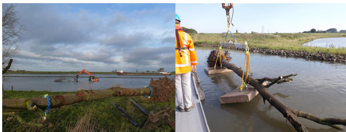
Figure 2: Entire trees were fixed in the riverbed and side channel (left) and concrete slabs were used to submerge the trees in deep erosion pits (right).
