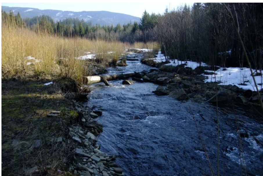
Figure 2. Downstream part of the restored reach with exposed log as a stabilization element (the log was originally at the channel bed level).
