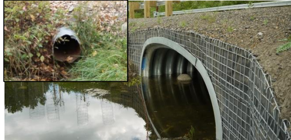
Figure 7: Culvert connecting alcove wetland before (inset) and after
