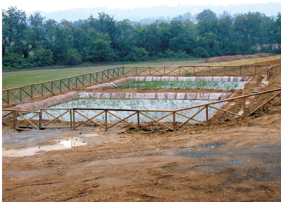
Figura 1 The constructed wetland realized near Sellustra stream
