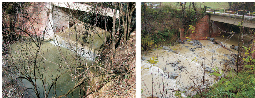
Figura 2 The slope built with stone block in order to smooth the drop under the bridge.
