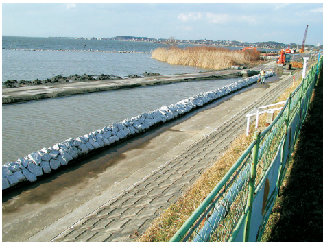
Figure 3 Lake Kasumigaura: Restoration of the littoral zone. Left: Banks are covered with concrete (during construction). Right: Recovery of natural vegetation (about three months after restoration) (Photos: K. Nakamura)
