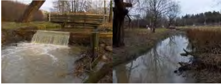
Figure 4 – The Matapuro dam and the stream before the restoration.
