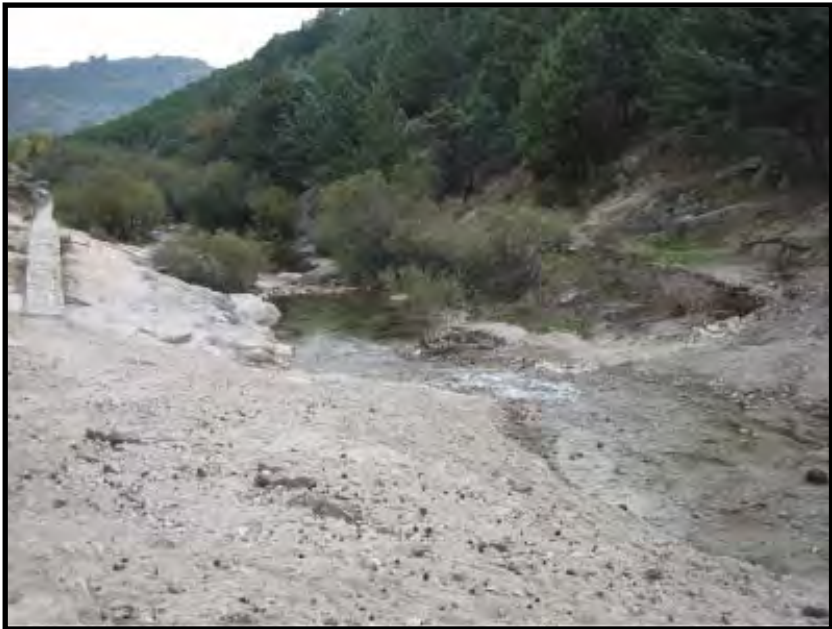
Figure 3 – Manzanares dam after the demolition
