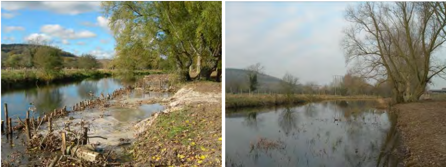
Figure 4 – Constructing an aquatic ledge at 7 hatches (left) and ledge fully submerged in winter
