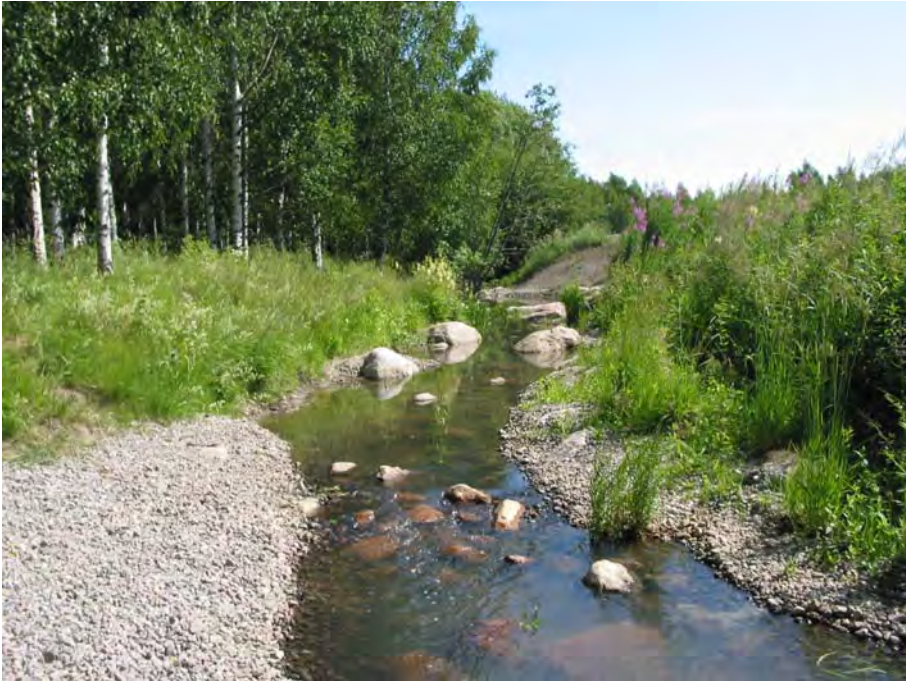
Figure 1 - The straightened Longinoja brook was restored with new slight meanders and stone material.
