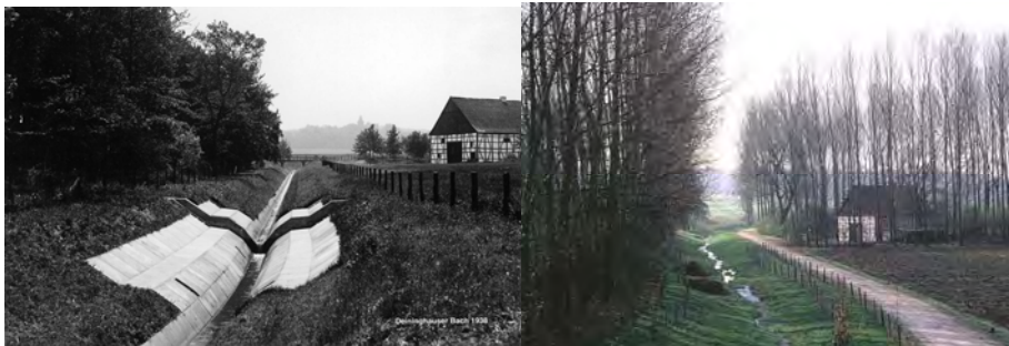
Figure 1 – Deininghauser Bach - Regulation in the upstream area 1938 and situation after restoration 2002;
