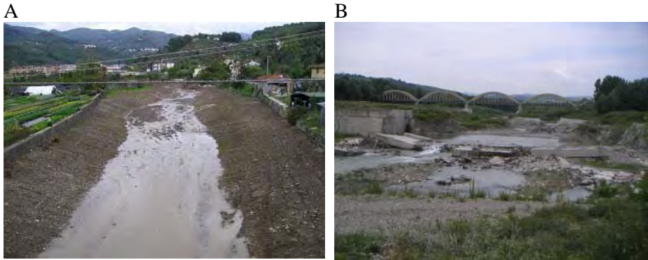
Figure 3 – Examples of degraded river conditions in Northern Apennine (Italy). A) Ombrone R.: common practice of channel maintenance by periodic clearing and dredging. B) Panaro R.: channel bed incised into the clay substratum.
