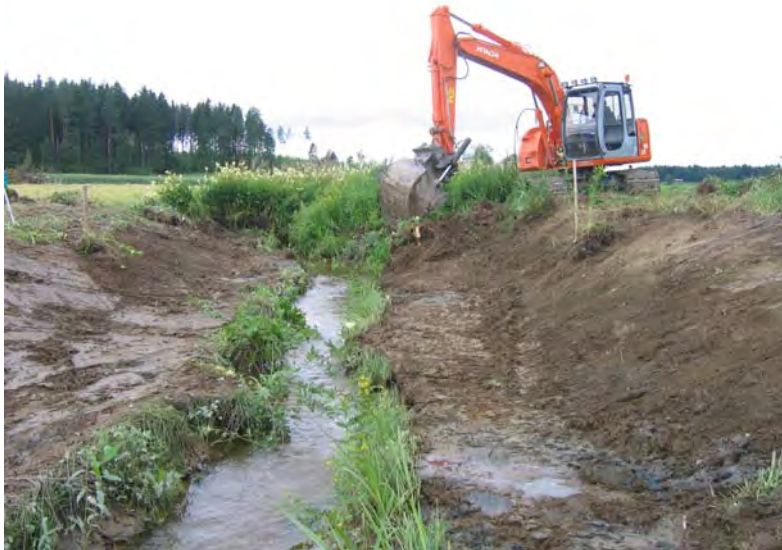
Figure 2 - In the two-stage profile of Juottimenoja brook the naturally enhanced bed was preserved as low flow bed. Only flood terraces on both banks were excavated. The bed is not affected and the water area remains narrow and deep enough for fish.
