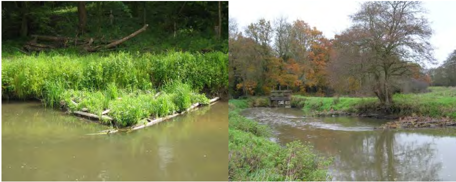
Figure 3 – Vegetated tree deflectors (left) and reduced impoundment (right) at Fovant
