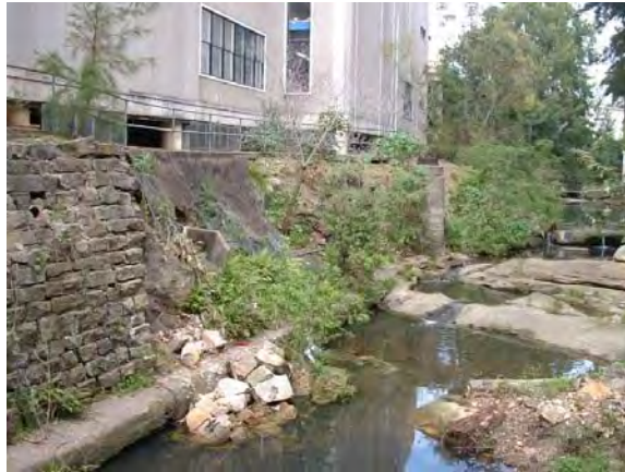
Figure 4 - Before: Looking upstream showing the left hand filled bank eroding and collapsing. Note the close proximity of the buildings to the bank.
