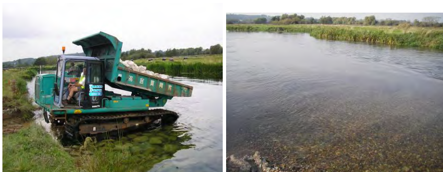
Figure 5 – Installing the stone base (left) which was then topped with gravel to create a spawning riffle at Hale
