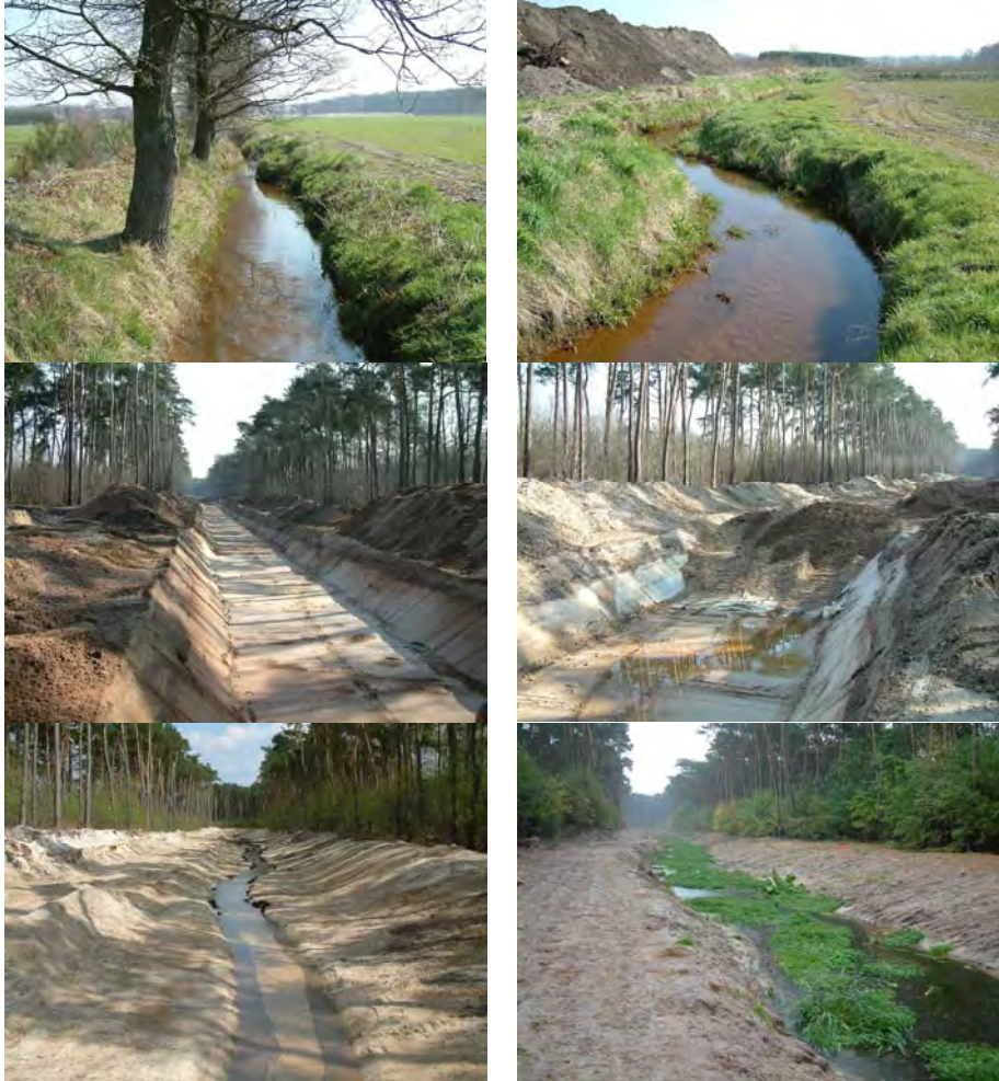
Figure 2 – Upper row (a and b): original reach of the Voorste Nete. Middle row (c and d): Excavation of a 5 m wide stretch for placing the bentonite mat and refilling with the original sand. Bottom row (e and f): Diverted reach of the Voorste Nete, dug out in sand filled bentonite lining with transferred substrate from the original reach, and the same stretch 6 months later during first monitoring showing the changes in dimensions caused by a summer storm in 2004.
