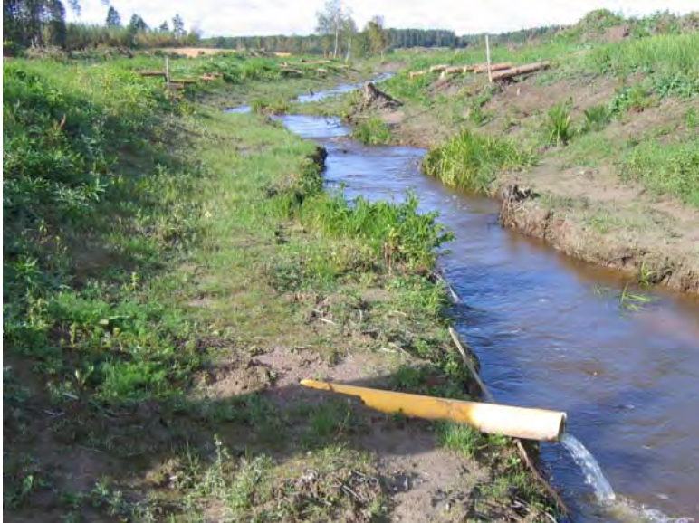
Figure 3 - Drainage pipes coming to the flood terrace in Juottimenoja brook. Herbal vegetation and roots of trees protect the slopes from erosion.
