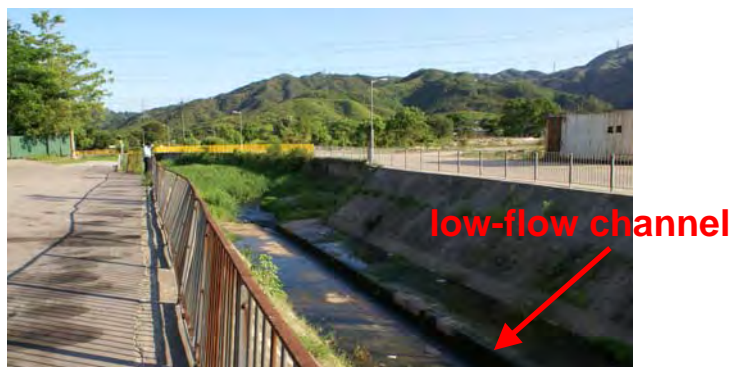
Figure 1 – A typical flood control concrete channel in Yuen Long, Hong Kong.
