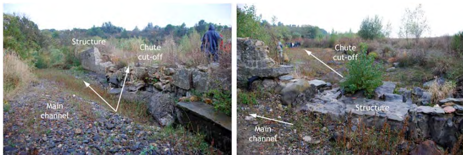
Figure 7 – Example of management for naturalness along the Clamoux River. The breach opened during the flood of November 1999 was artificially increased to force the river temporarily to cut-off the meander during the next floods.
