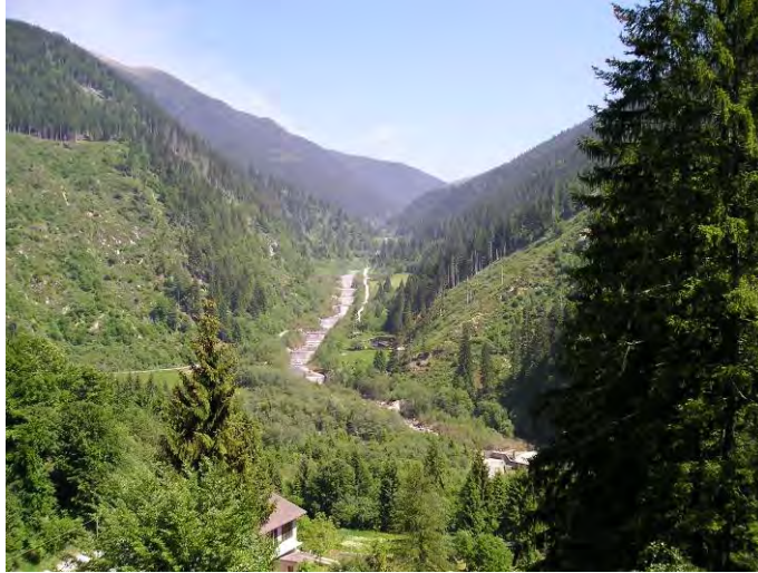
Figure 1 – Looking upstream to the Maso di Spinelle catchment. The tall check-dams built in the 1980s are visible in the channel.
