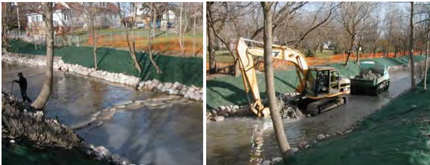
Figure 3 - Arcuate rock ribs across the channel (left) and digging of pools within the project reach (right).
