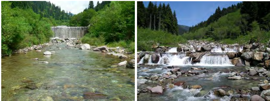
Figure 2 – Different torrent control works in the Maso di Spinelle river: “traditional” reinforced concrete check-dams (TR, left) and “artificial steps” (AS, right).
