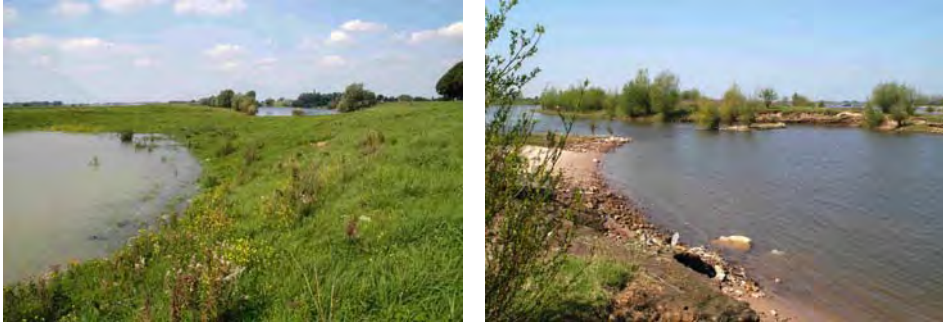
Figure 3 – Bislich-Vahnum proposed site for side channel (left) and implemented side channel near Gameraen along the river Waal (right)
