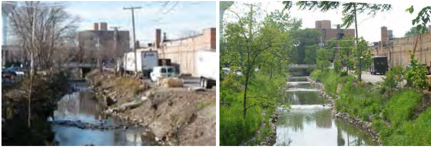
Figure 1 - West Branch of the North Fork of the Chicago River in downtown Northbrook showing conditions before (left) and after (right) naturalization.
