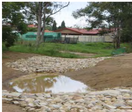
Figure 3 - During works: Looking upstream along the same reach at the completed rock ramp bed controls. The permanent ponds are starting to fill. Riparian zone replantings are yet to commence.
