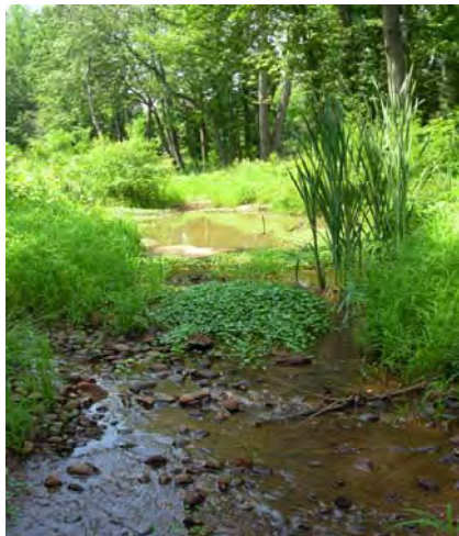
Figure 3 - Photo of a Coastal Plain stream in Annapolis, Maryland USA after it has been re-designed to accommodate higher flows and remove pollutants.
