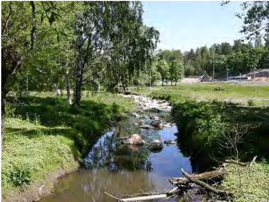
Figure 5 – The Matapuro stream after the restoration, low flow condition.
