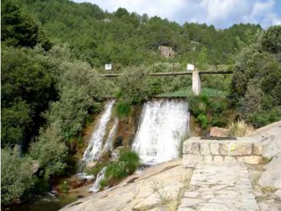
Figure 1 – Manzanares dam before the demolition
